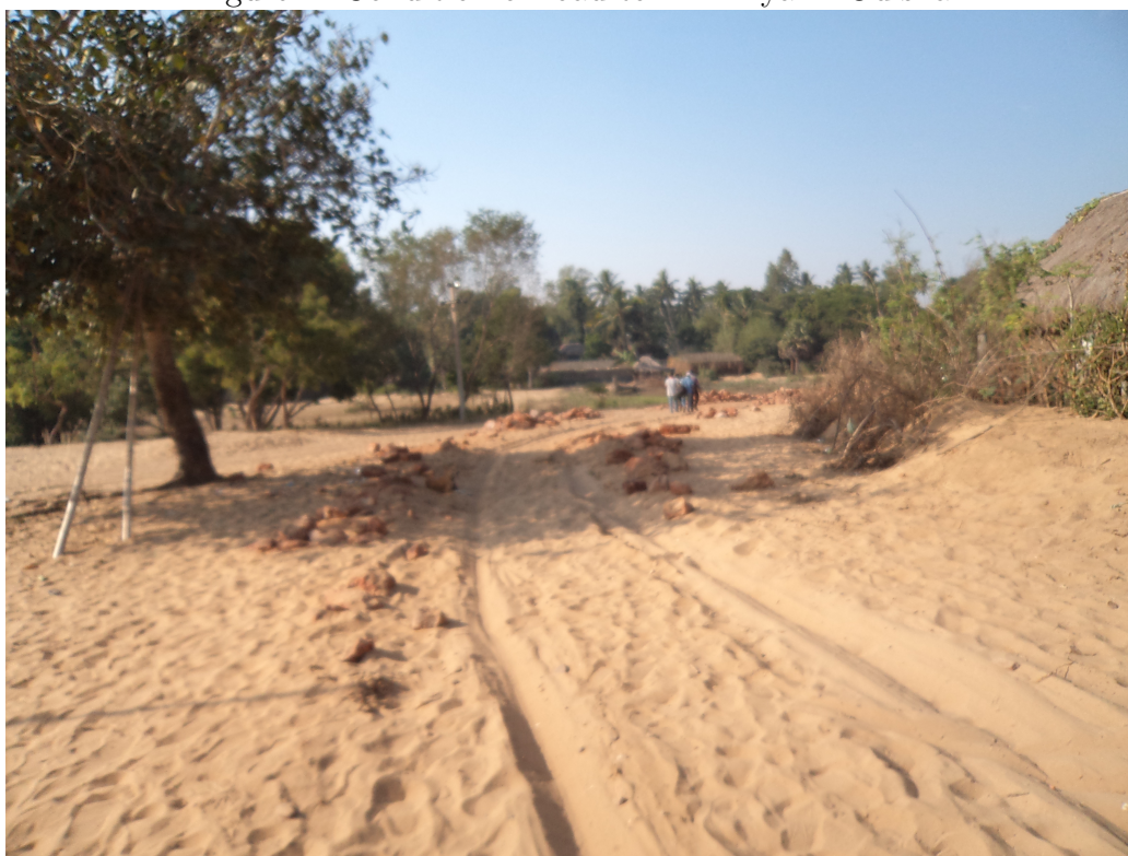
Figure 2: Condition of road to Dhinkiya in Odisha
